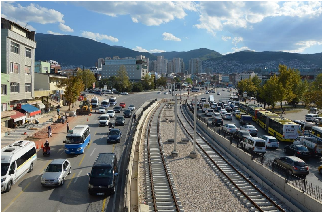
Figure 4. T-2 Tram line of Bursa [5]
