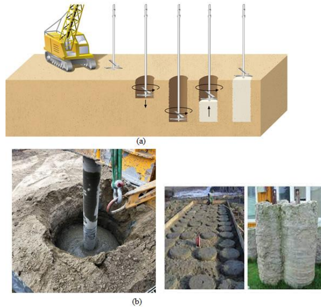
Figure 1 (a) DSM processes (b) Some constructed DSM columns
